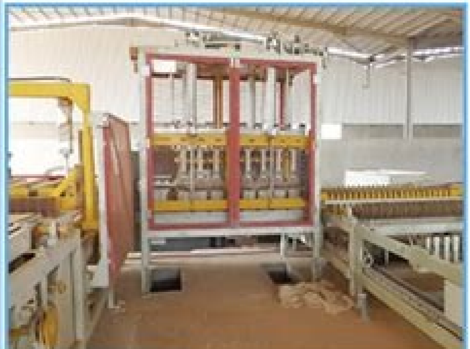
Grouping system installation
