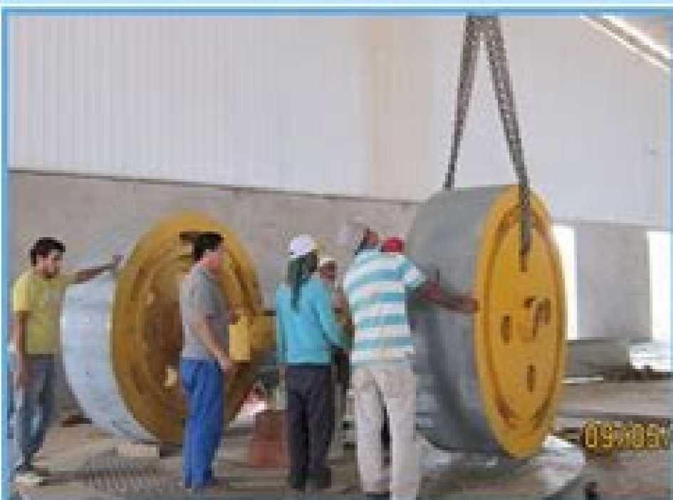
Wet pan mill installation
