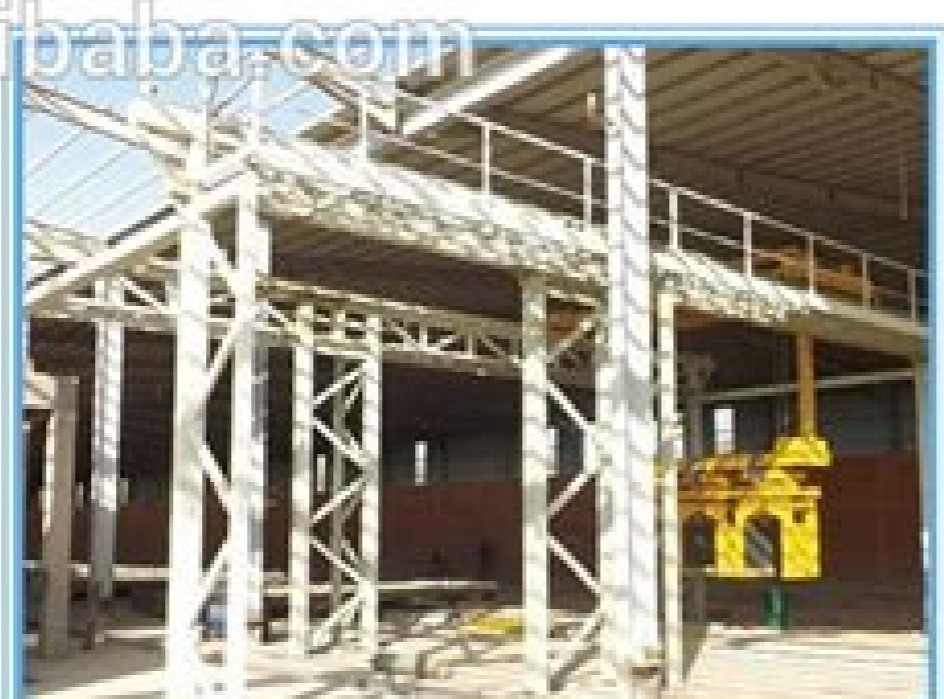
Brick unloading machine installation
